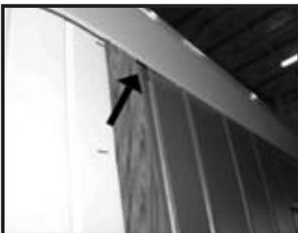
7. When Installing the panel, ensure that it is completely inserted in the top channel. Then follow the removal steps in reverse order.
