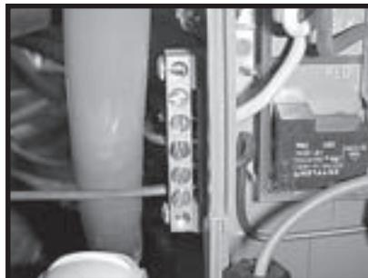
A grounding lug has been provided on the exterior of the control box to allow connection of a ground wire to a local grounding point in compliance with the National Electric Code (NEC) and all local codes.
