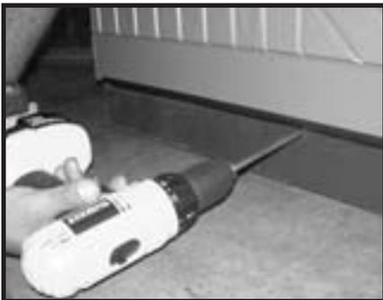
5. Remove side bottom screws leaving the center one for last. Remove center screw while supporting panel in place
