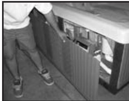
6. After the center screw is removed, the panel will slide down, then remove panel.
